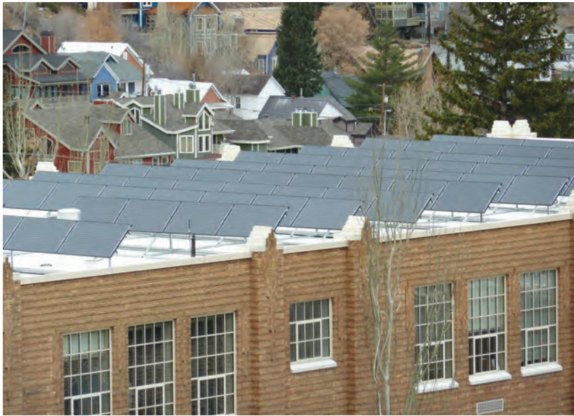
Park City, Utah, installed a PV system on its city hall building in 2010. This system provides enough electricity for three average Utah homes and saves the energy equivalent of burning 23,000 pounds of coal each year.
