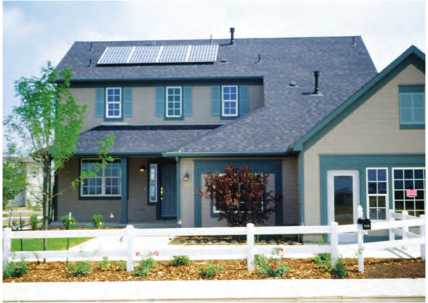
Figure 2.6. This rooftop system in Longmont, Colorado, meets about 25 percent of the household's electric needs and provides back-up power to critical appliances during utility power outages.
